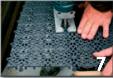
Cut boards to the required shape with a jigsaw...
