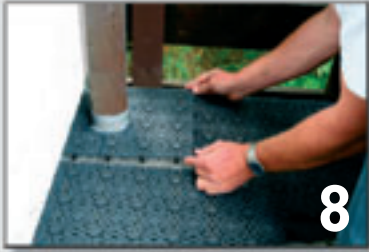
...to fit curves and feed-throughs.
