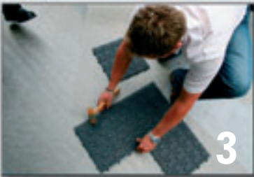
Join Enkefloor floorboards to form larger units.
