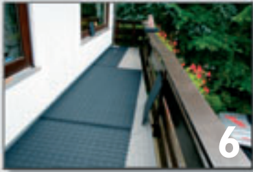
... insert an expansion strip after approximately 4 to 8 board units.
