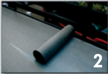
Roll out Enkefloor-fleece to prevent mechanical damage.
