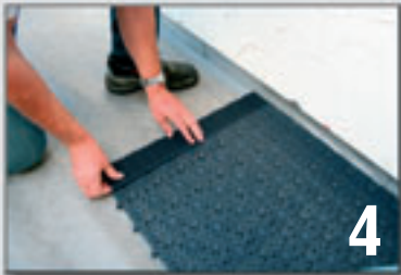
Lay floorboards allowing a gap of 5-10 mm between floor covering and wall.
