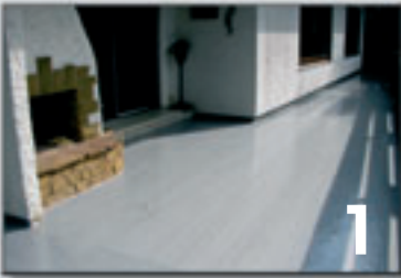
Clean the floor, apply Enkopur sealant and allow to cure.
